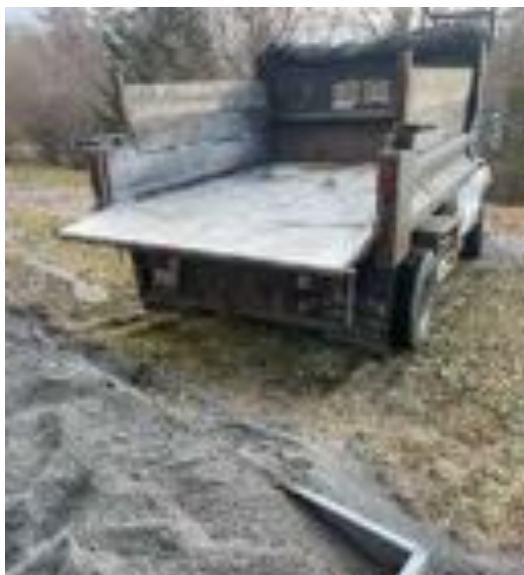
Stone dust was dumped into the frame base.
