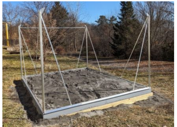
The frame corners are in place.
